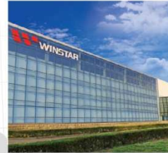
LCM Facility Jiang Su, China
